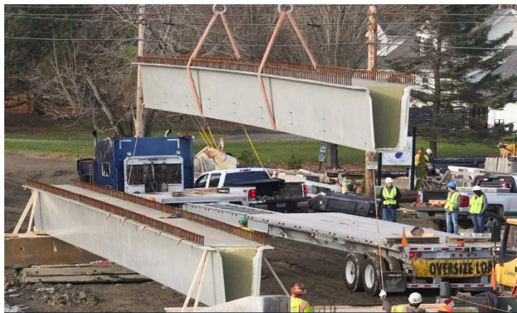
Figure 5 – Composite GBeams Fabricated by AIT.
